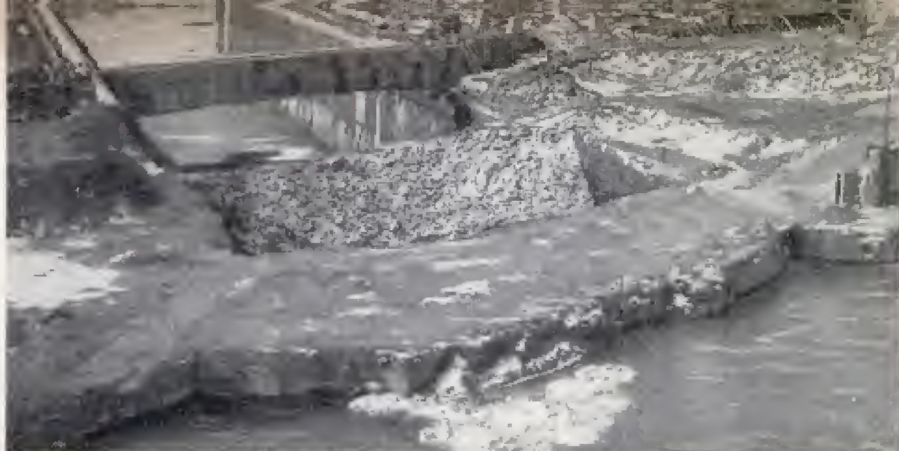
Rock plug separating forebays was loaded with 12,000 pounds of explosives. Power station was 160 ft. distant
